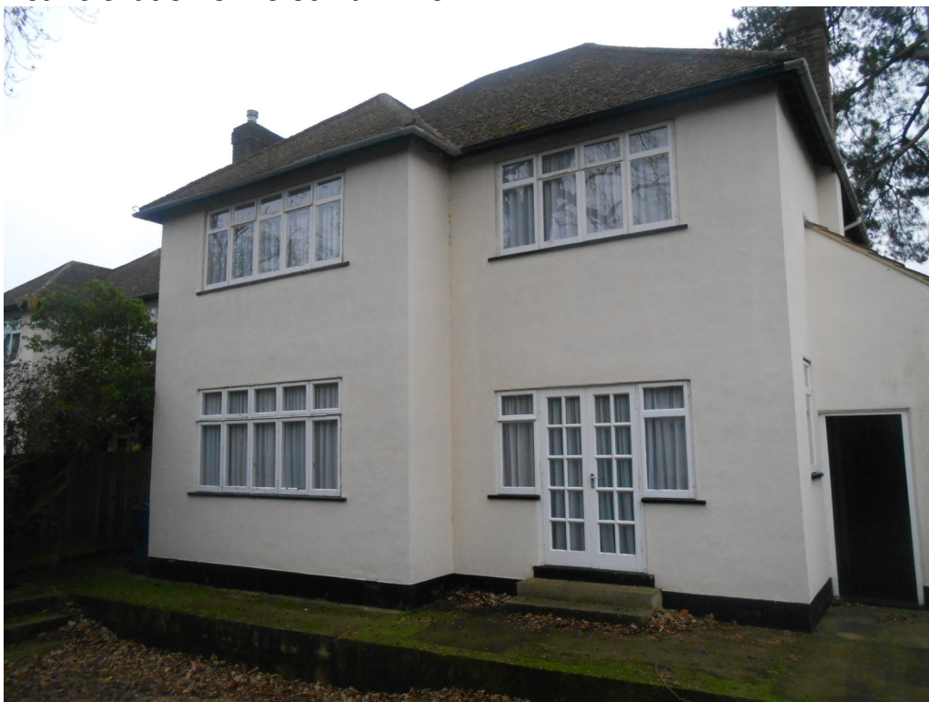
Rear elevation of no 30 Park View
